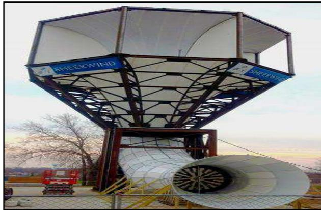
Fig.16 Invelox wind power generation technology
